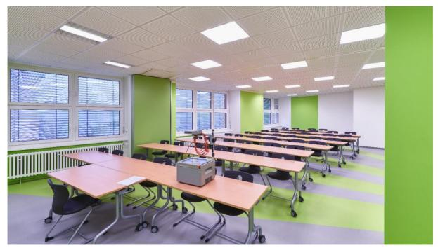
Field of application: Gypsum board ceiling | perforated gypsum board ceiling tile with integrated capillary tube mat OVAMAT, heating and cooling function
